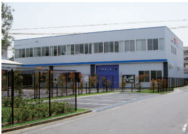
工場新築工事
